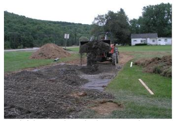
road fabric and applied stone right up to the highway. On the north entrance we just did stone. For the driving lane that runs parallel to Route 38, we took off the sod, laid fabric, and dropped gravel for about 100 yards. We also put in a gravel pad for the dumpster.
